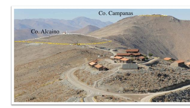
Figure 12: Photo of Cos. Alcaino (foreground) and Las Campanas (background). The amount of earth removal necessary for GMT is indicated in yellow
